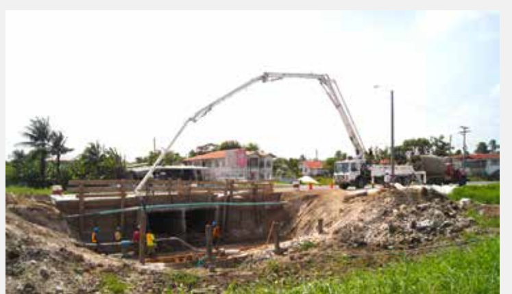
CONSTRUCTION OF HIGHWAY BRIDGES & FOUNDATION
