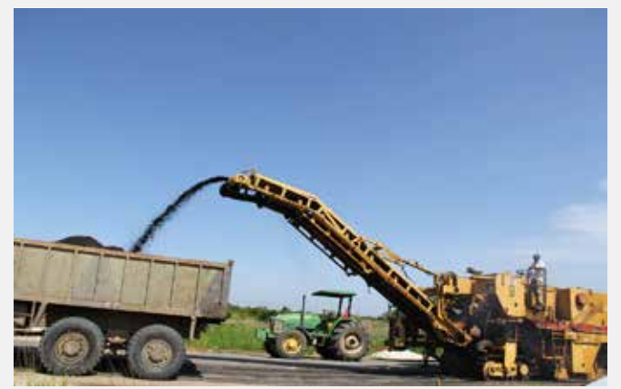
HIGHWAY CONSTRUCTION & PAVING
